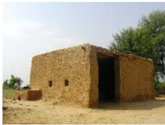
Figure 4: Example of a cubic simple house (Simple House I): a mud house in a local village in Pakistan.
